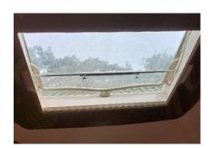
Some HEKI rooflights are prone to being blow open when the wind is strong and from the wrong direction. The Windjammer cures this problem.
